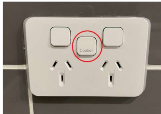
If applicable electric cooktop isolation switch located in kitchen
