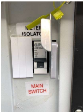
Main Switch shown in the ON position
