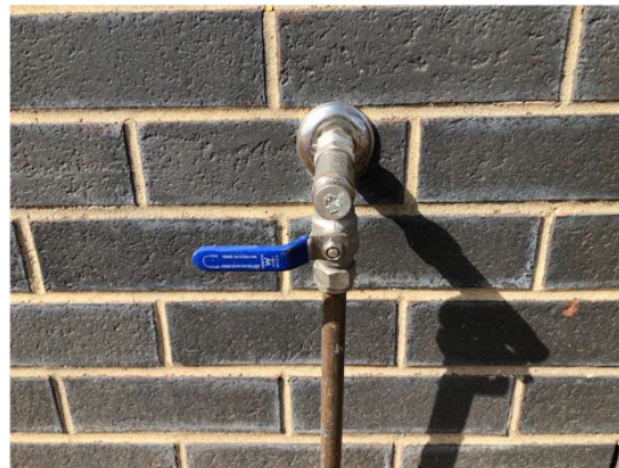
Water valve shown below in the OFF position
