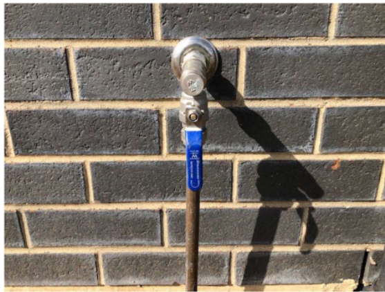
Water valve shown below in the ON position
